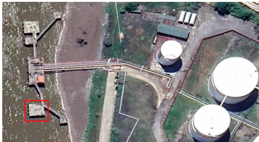
Fig. 1. Berthing structure (red box) for LNG terminal (Source: Google Map).
